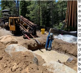
from now into the future and improve the ease of operations and maintenance activities. order to minimize disturbance to the Highway and Truckee River bed, the District chose to construct the project using Horizontal Directional Drilling which greatly minimized the environmental and traffic impacts of the project (horizontal drilling equipment pictured at left). This method steered a drill bit across and below the highway and river bottom to produce a small diameter pilot hole which is then
